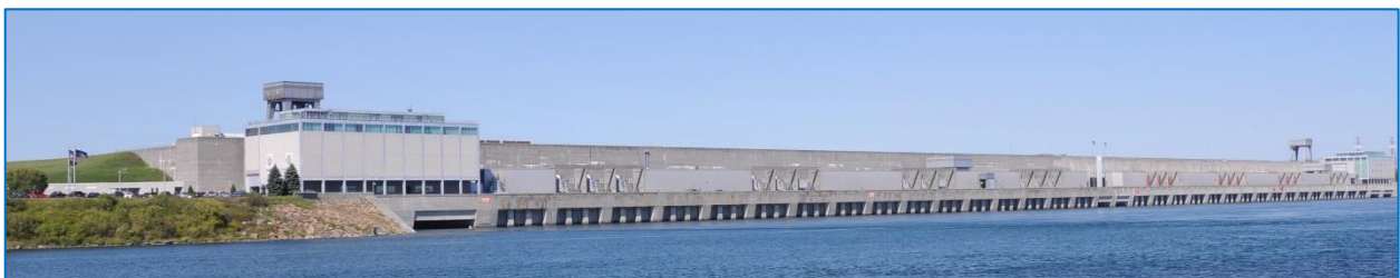
New York Power Authority
