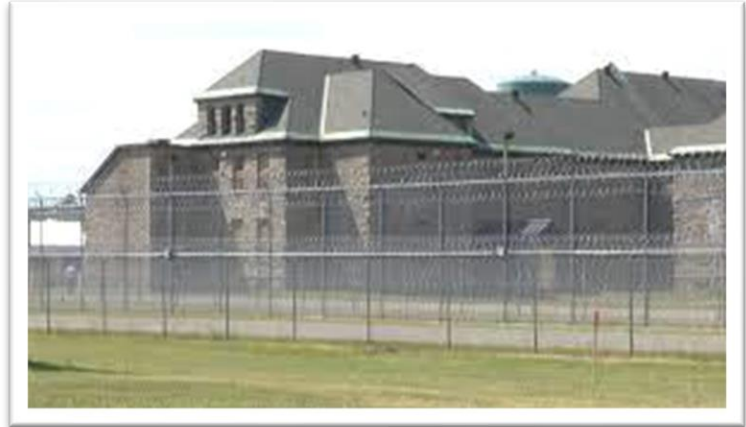
The recently closed Ogdensburg Correctional Facility
