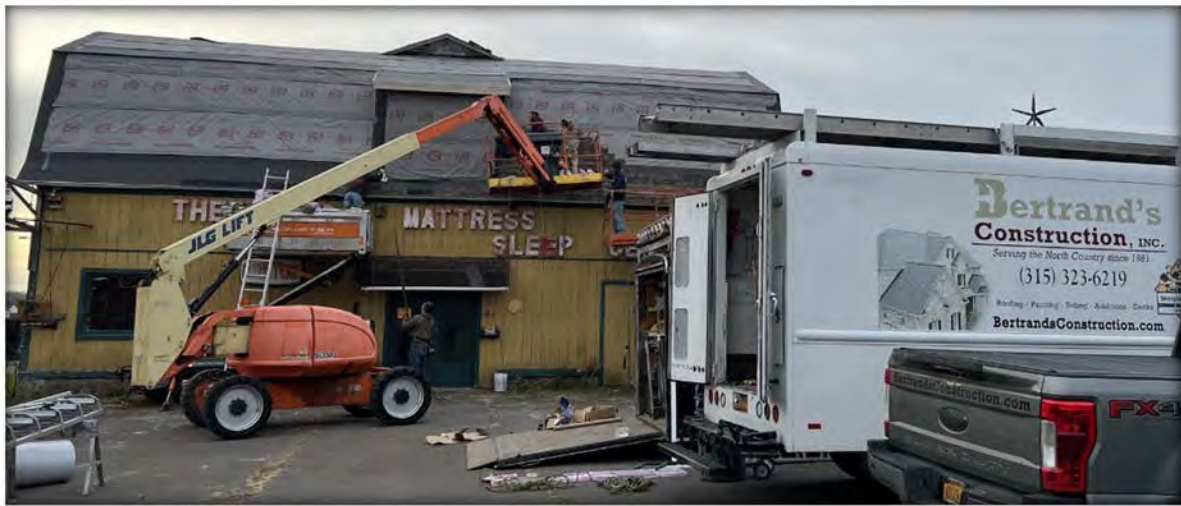
Construction underway at the future home of the Bent Beam Brewery in Canton
