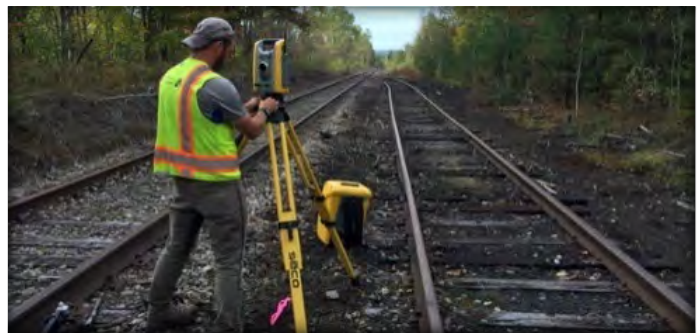
Photo Courtesy of Erdman Anthony Consulting Engineering Firm
