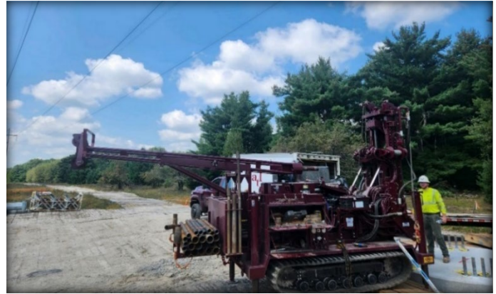
ATL's CME rubber track drilling rig
