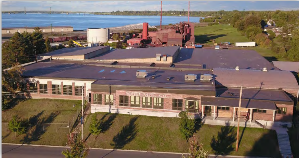
100 Paterson Street Facility, Ogdensburg
